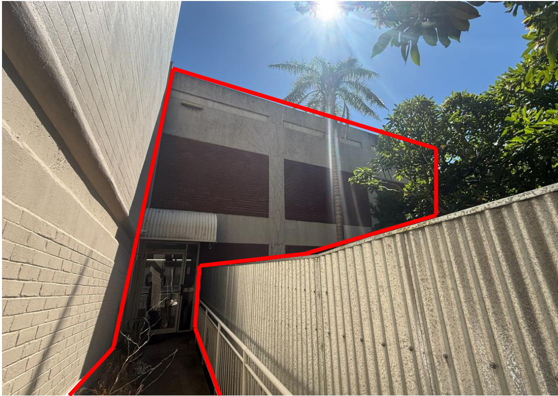
Figure 3: View west of existing building entrance and eastern facade
