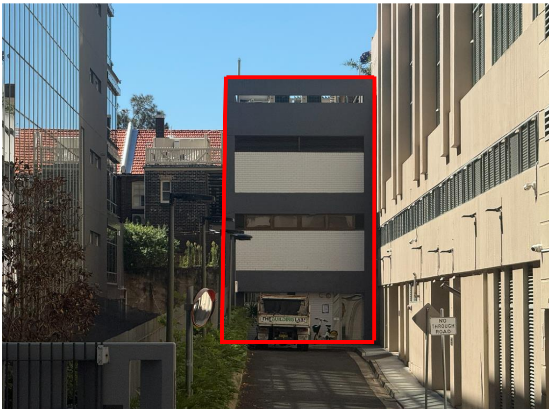
Figure 4: Site viewed from Jenkins Street/Southern elevation
